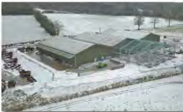
ScanStone's new building.
